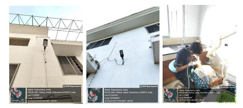
Sensor based lights convert light energy to an electrical signal output. They can detect the amount of light in a room or in an outdoor environment and raise /lower the blinds or switch on/off the lights automatically to improve the comfort level of the user thus conserving the electrical energy.
